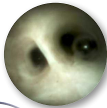
View of normal ducts
